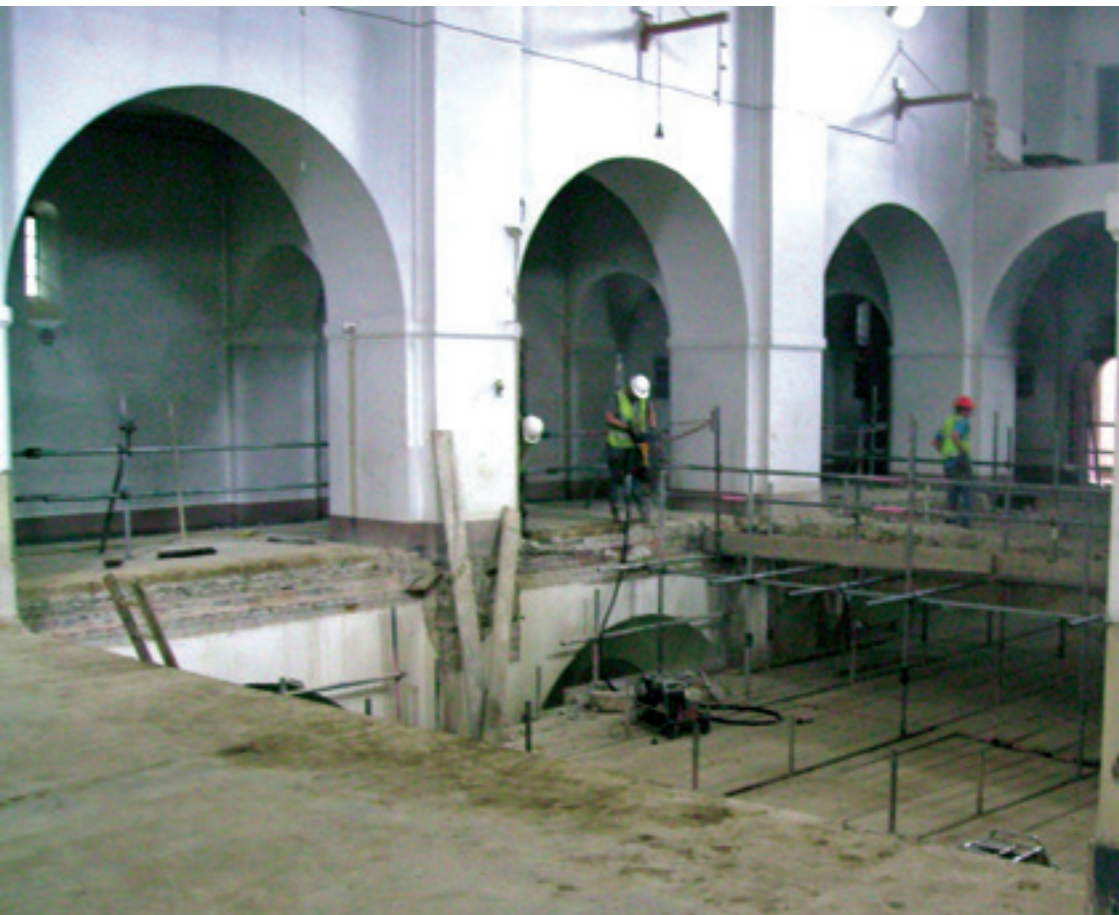
The floor being removed between Upper and Lower church
