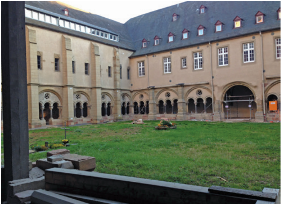
The Abbey cloister, in the midst of renovation
